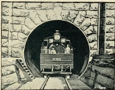
TUNNEL ENGINE EMERGING FROM PORTAL.
